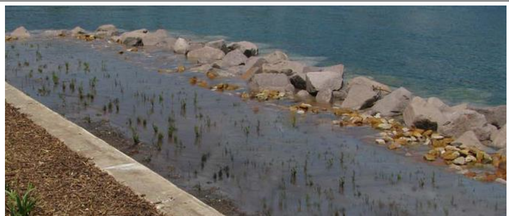
Constructed saltmarsh zone
