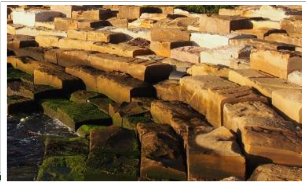
Sandstone block stairs/seating
